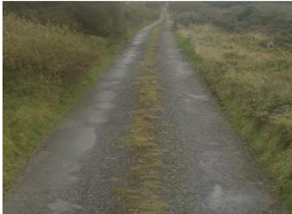
Plate 2 – Typical Local Road
